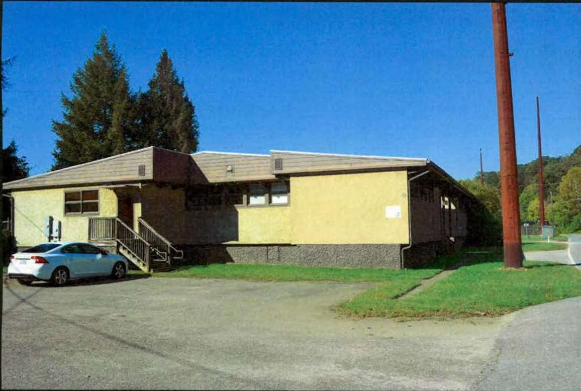
27. Buildings, 91 Thompson Street, 1956
