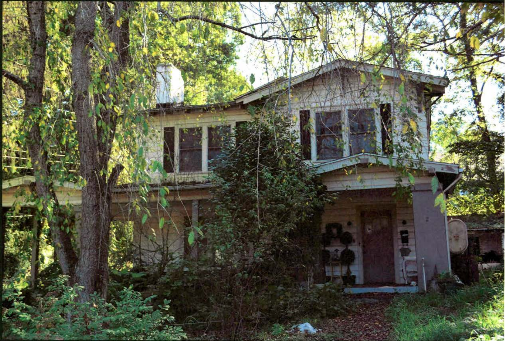
28. Harrell House, 2 Finalee Avenue, 1925
