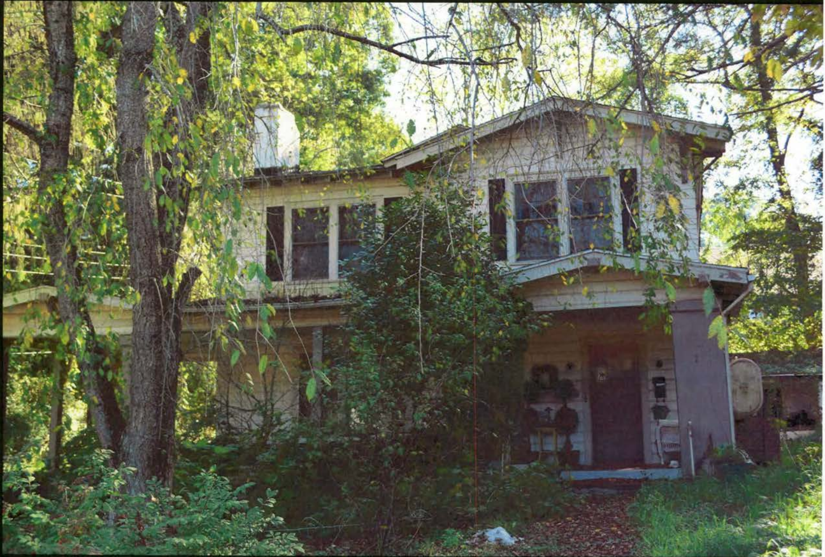
28. Harrell House, 2 Finalee Avenue, 1925
