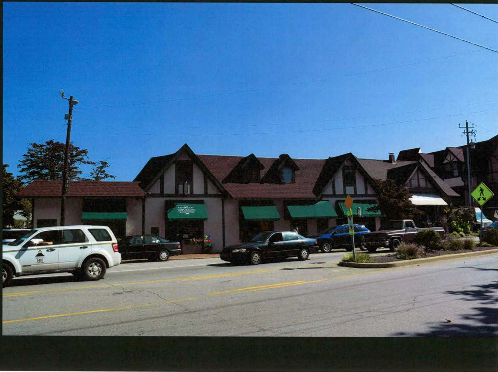
48. Biltmore Village Post Office (BN0153), 2 Brook Street, 1927
