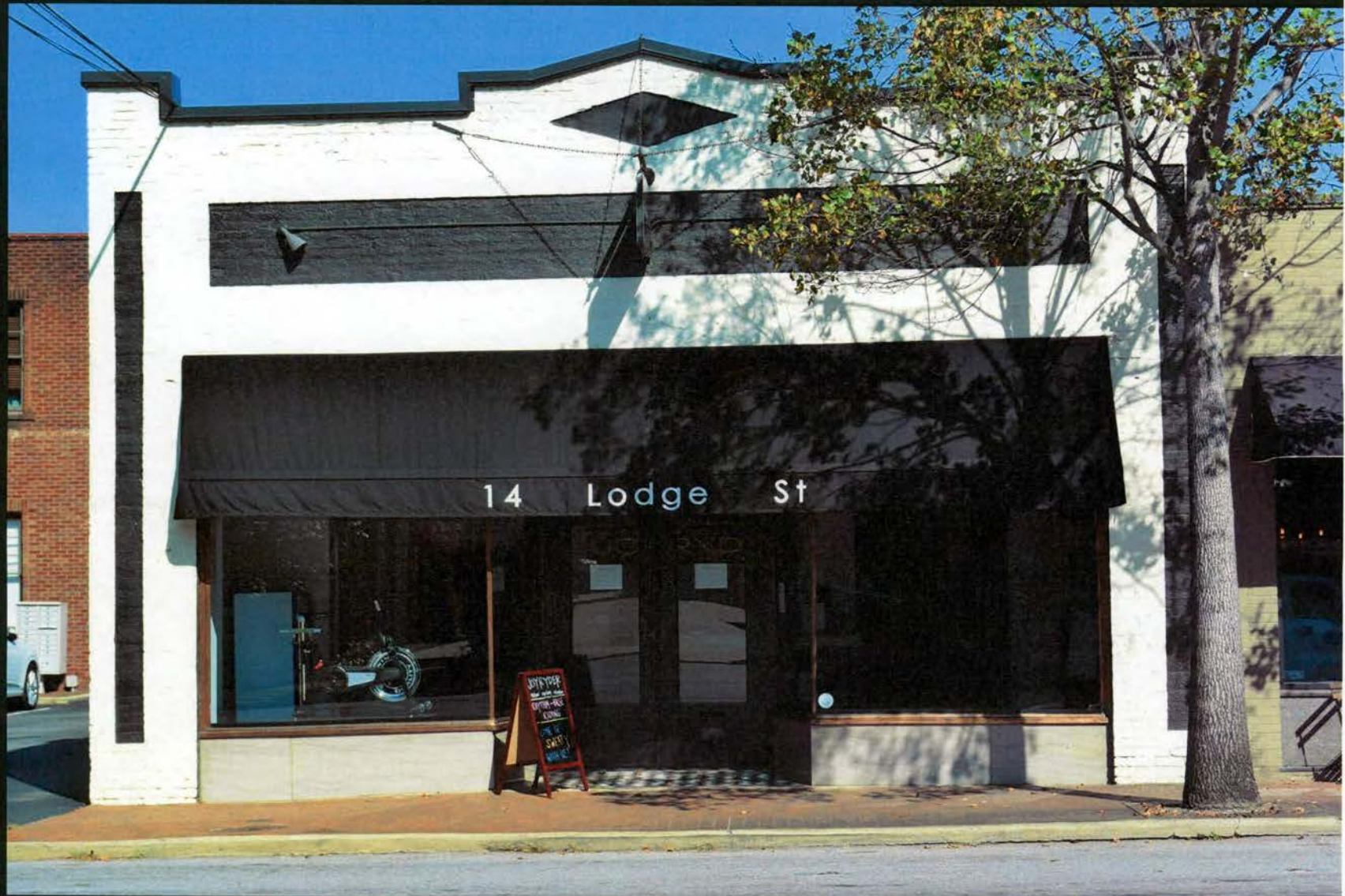
53. Building (BN5550), 14 Lodge Street, 1931
