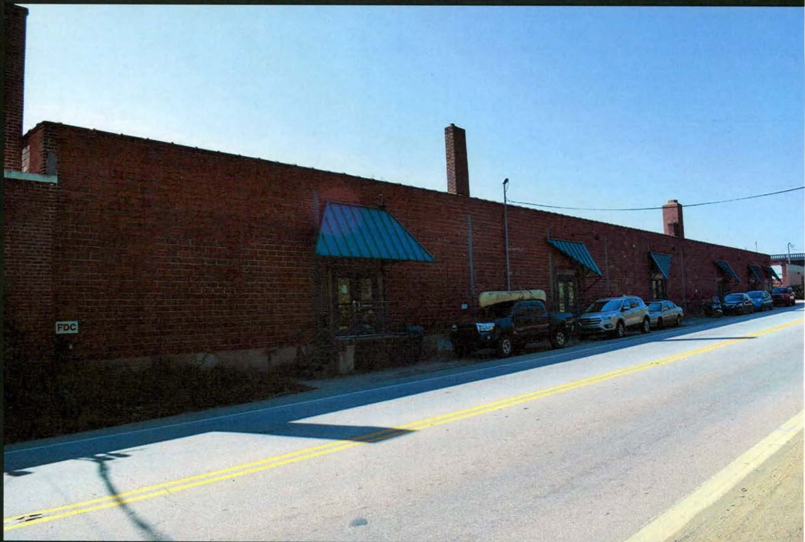
46. Habitat for Humanity, 31 Meadow Road, 1947
